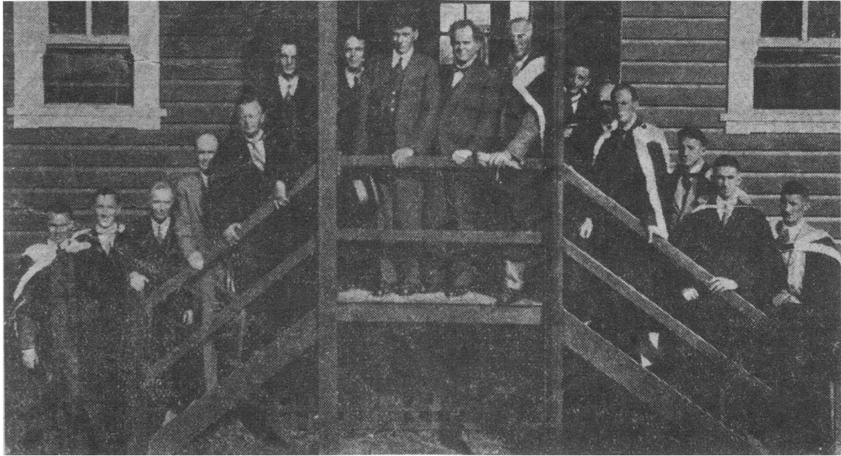
Opening of new school hall. The hall had been built by the students under the direction of Mr Les Pinn.
